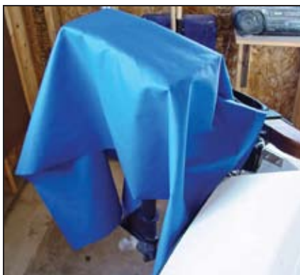
SurLast draped (wrong side out) over the cardboard pattern.
