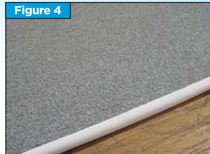
Finished carpet edge bound with a facing.
